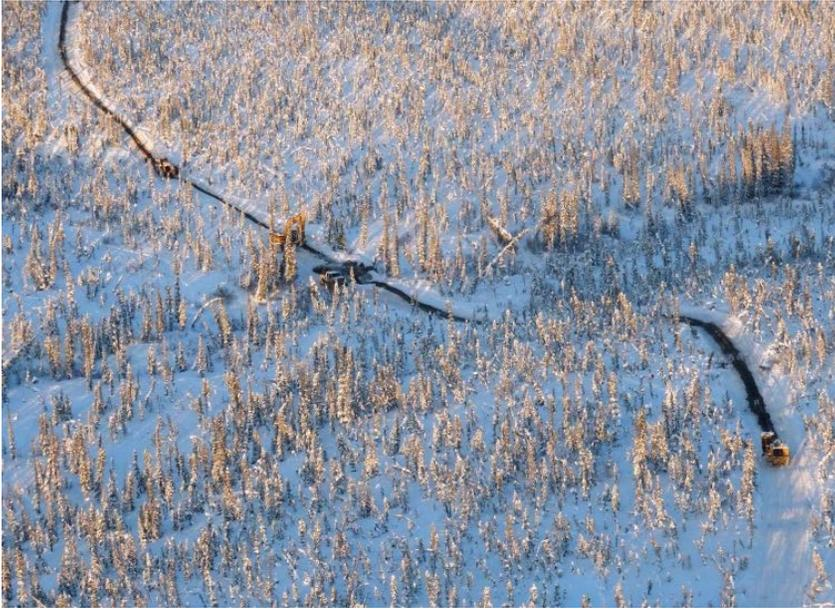
Aerial view of a saw, an excavator, and cable plough performing trenching and cable installation work.
